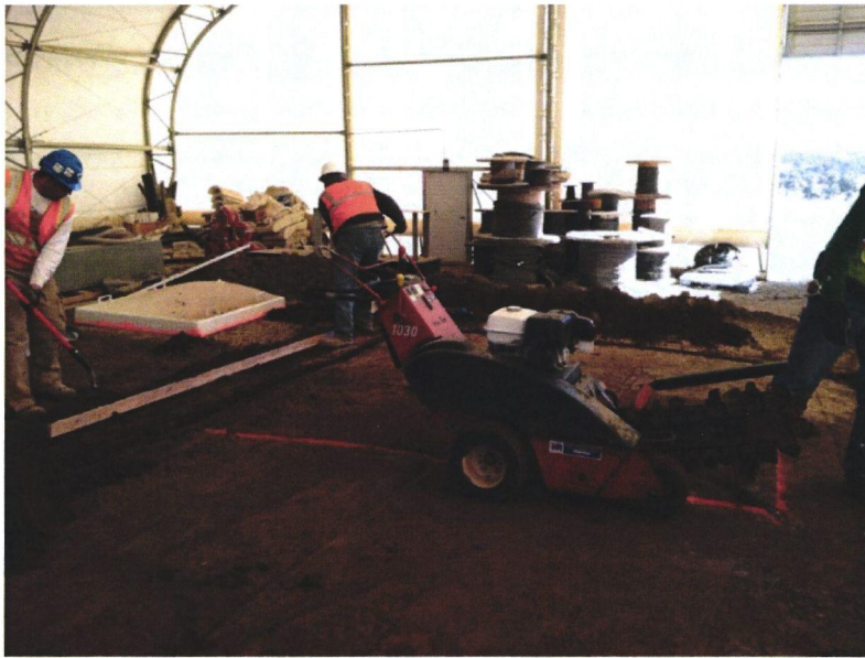
Figure 12 – Excavation of the outer trench using a trenching machine
