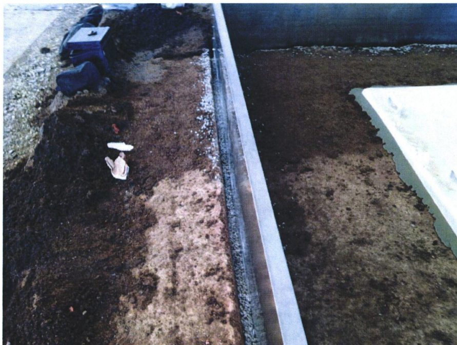
Figure 14 – Bentonite chips placed along the outside of the outer ring
