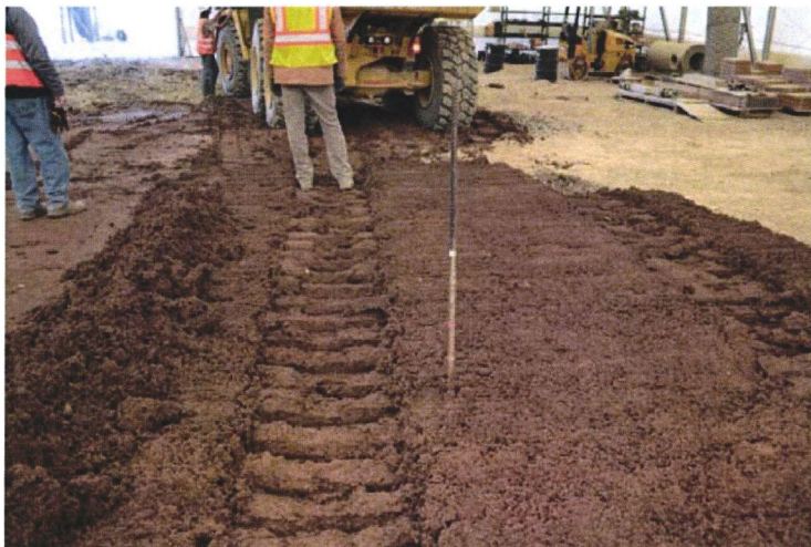
Figure 9 – North side lift 1, 12 inch loose
