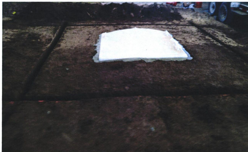
Figure 13 – Inner ring set in place with the excavated outer ring trench.
